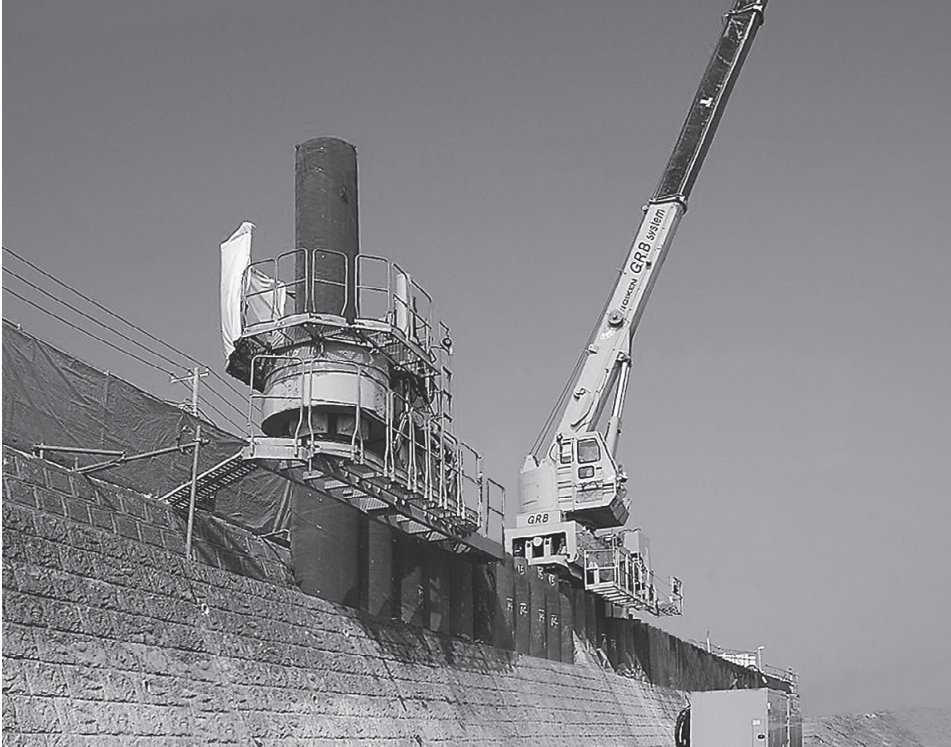
An Implant Levee under construction in Kanagawa Prefecture GIKEN LTD.
