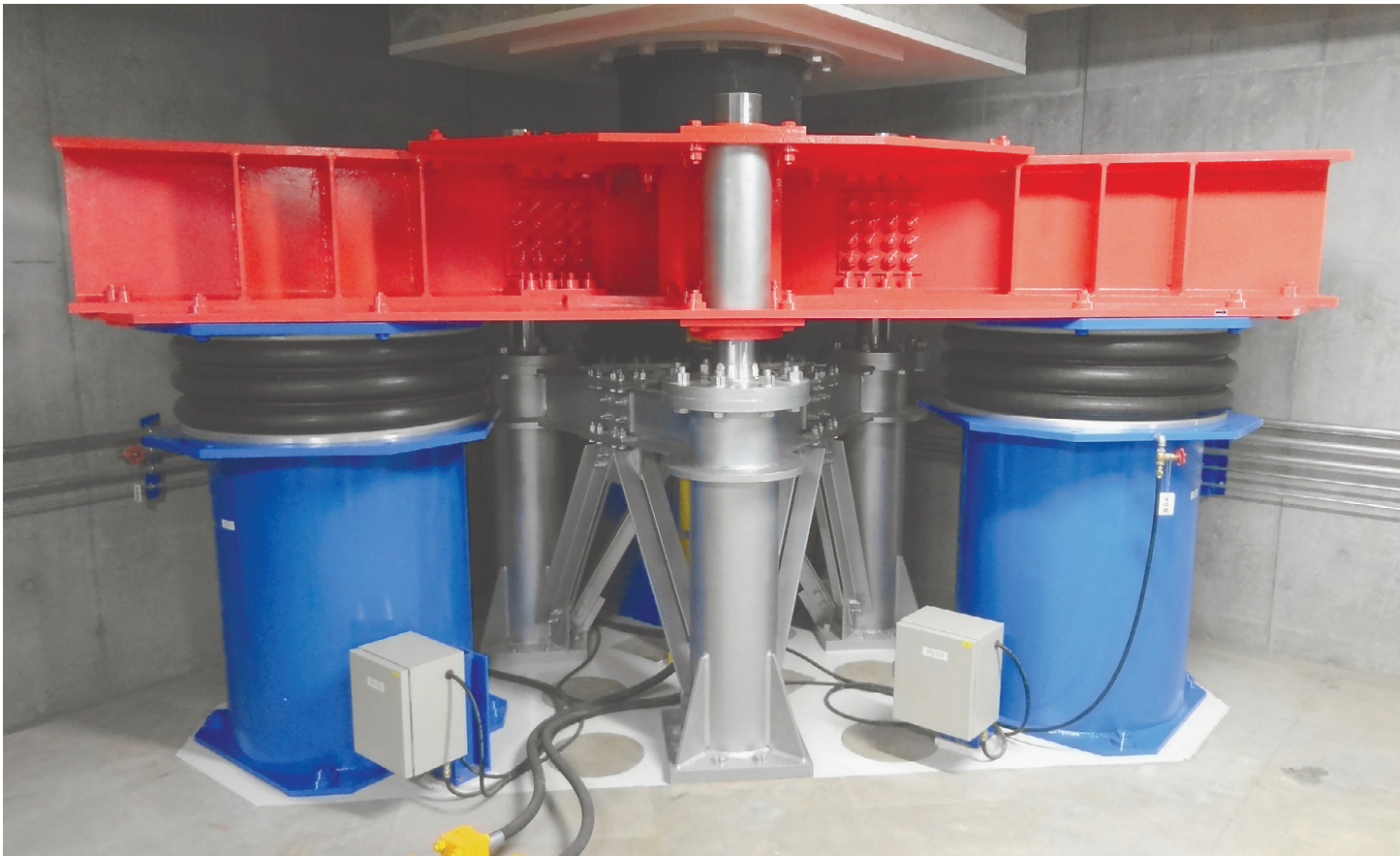
Seismic isolation systems are placed underneath structures to cushion earthquake ground motion with rubber, oil or other substances. KOZO KEIKAKU ENGINEERING INC.
