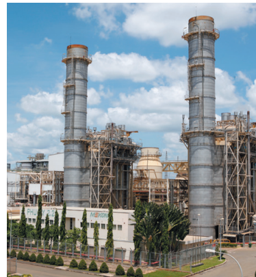
Phu My 2.2 , part of the Phu My Thermal Power Plant Complex, in Ba Ria-Vung Tau Province, Vietnam MECO
