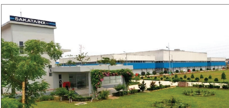
Sakata Inx India's Bangladesh Plant, commissioned in 2021, is a state-of-the-art facility that produces liquid inks for the flexible-packaging industry.
