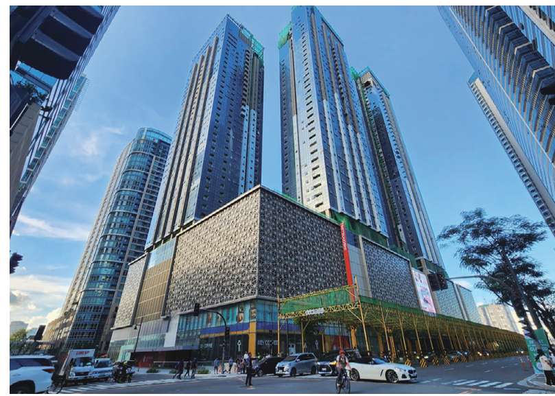
The Seasons Residences is a mixed-use development by Federal Land in collaboration with partners Nomura Real Estate Development Co. and Isetan Mitsukoshi Holdings Ltd. in Bonifacio Global City, the prime business district in Taguig. Its four residential towers, anchored by shopping mall Mitsukoshi BGC, integrate the Japanese traditions of innovation and excellence with Filipino hospitality and sense of community.
