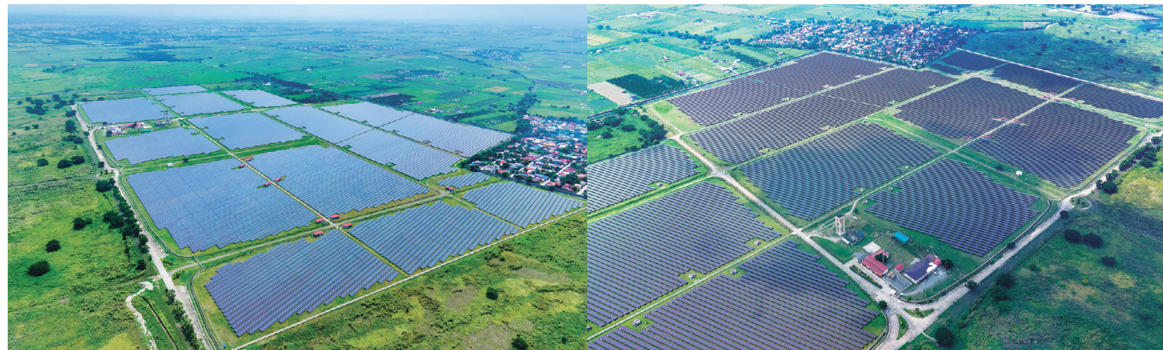
The 70-megawatt Tarlac Solar Power Facility in Tarlac is owned and operated by YGC's PetroSolar Corp.
