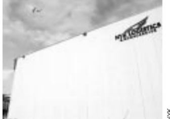
The headquarters of NYK Logistics Iberica in Barcelona
