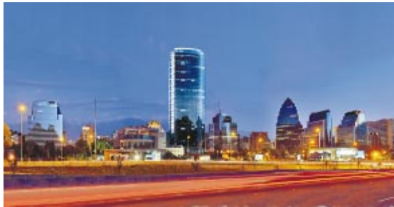
The Titanium La Portada Building will be the landmark of Santiago, the capital of Chile, and will change the entire skyline of the city.
