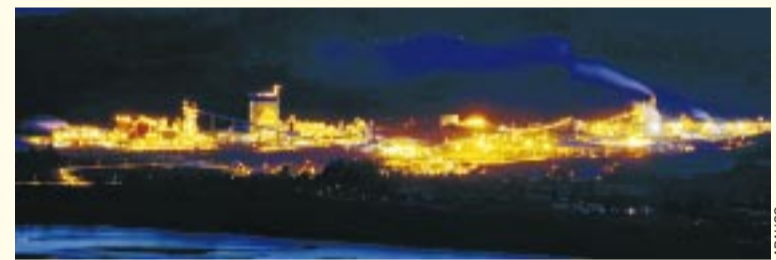
The Nueva Aldea Forestry-Industrial Complex in Nuble province — with its wood pulp mill, log merchandiser, the largest sawmill in the country, a panel mill and two cogeneration facilities for clean energy — positions the Chilean forestry industry at a level of excellence in the world.
