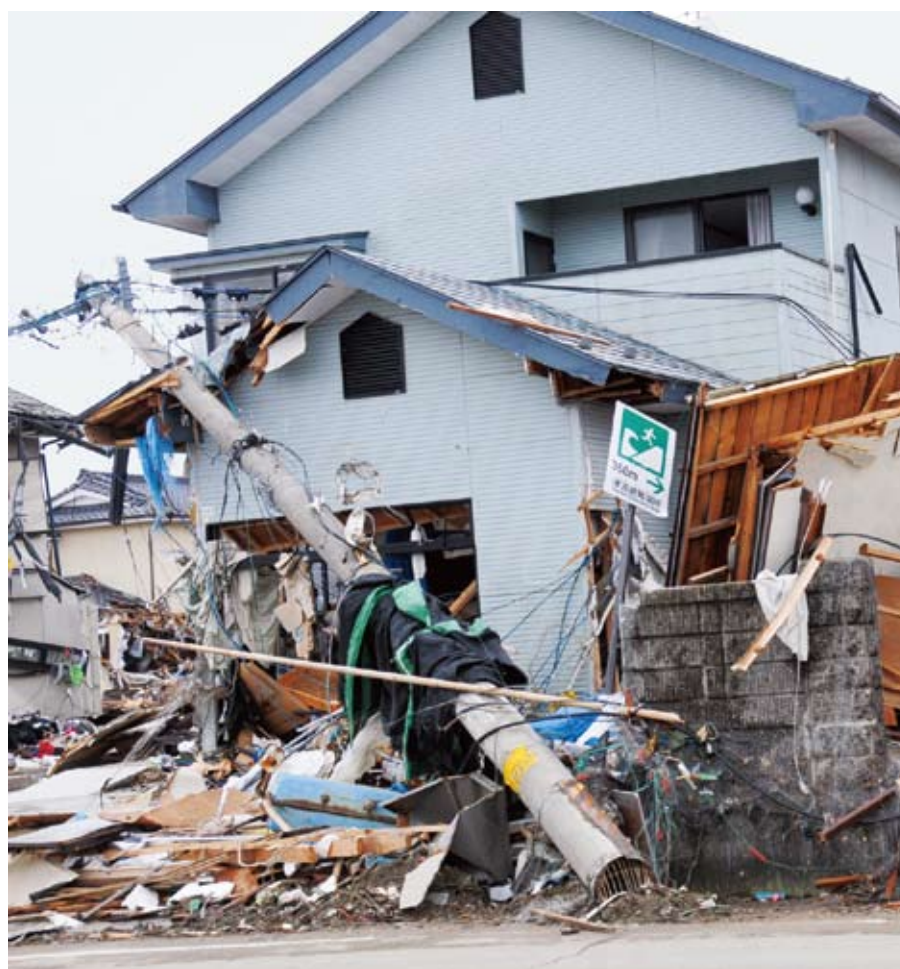
Unlivable: Houses damaged and destroyed by the March 11 tsunami are seen in Shichigahama, Miyagi Prefecture, on March 31.
