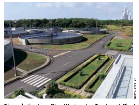
Through the Juan Diaz Wastewater Treatment Plant, Nippon Koei LAC helped Panama City, one of the world's fastest-growing cities, meet its infrastructure needs.
