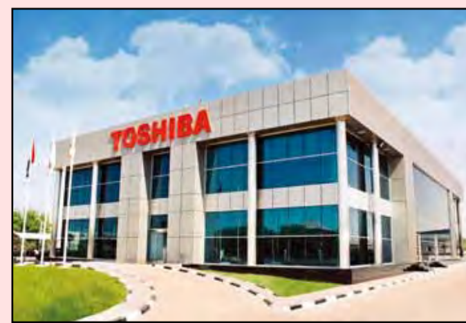
Toshiba set up a showroom and headquarters for the Middle East region in the Jebel Ali Free Zone in Dubai.
