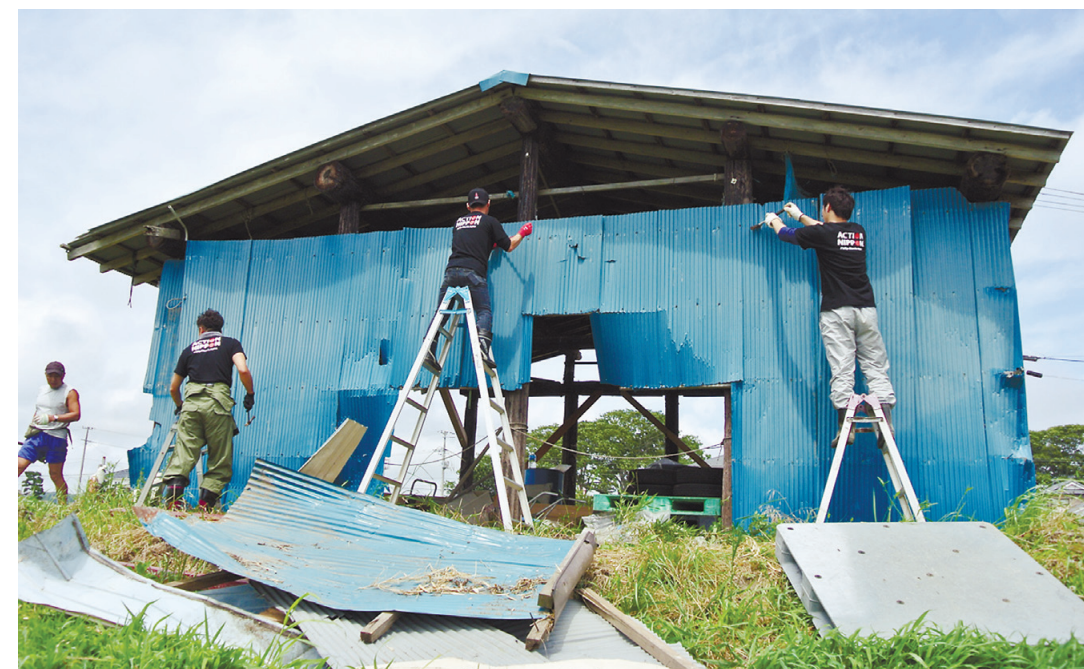
Rebuilding a storehouse at Yotsuba Farm, Higashi-Matsushima 東松島、よつばファームでの倉庫の修理 PHILIP MORRIS JAPAN
