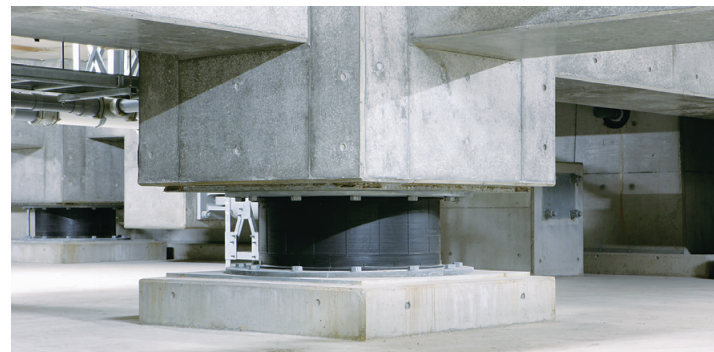
Seismic isolation equipment 免震装置 STARTS CAM
