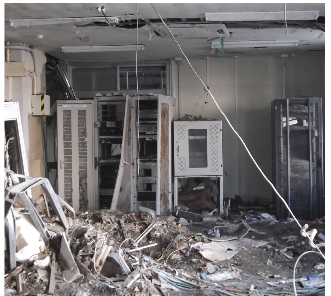
A server room severely damage in the earthquake and tsunami in Rikuzentakata, Iwate Prefecture. RIKUZENTAKATA CITY
