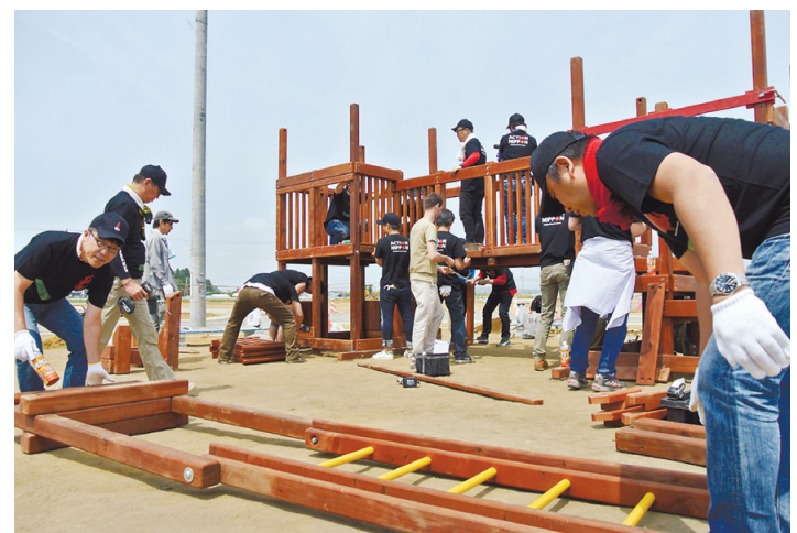
Building a playground at Aoi Area, Higashi-Matsushima 東松島、あおい地区での遊具設置 PHILIP MORRIS JAPAN
