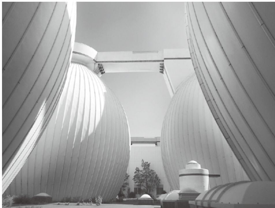
These large tanks in Yokohama City process sludge from sewers, extracting methane gas that can be used for fuel. YOKOHAMA CITY
