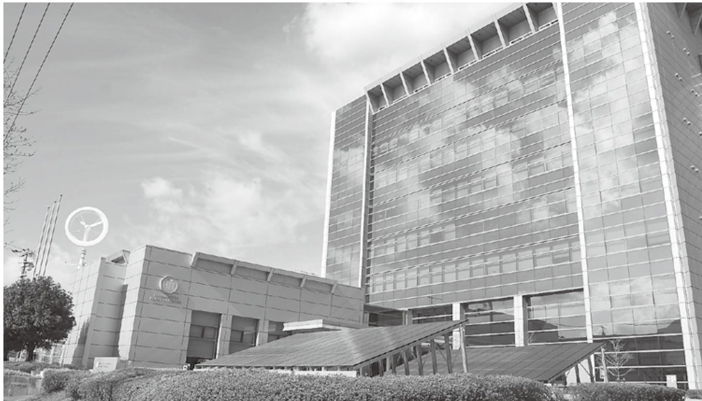
This Kitakyushu office building houses a community energy management system, or CEMS. KITAKYUSHU CITY
